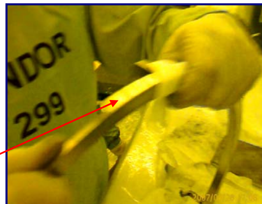
Fig 61: Wiping down entire lift ring
